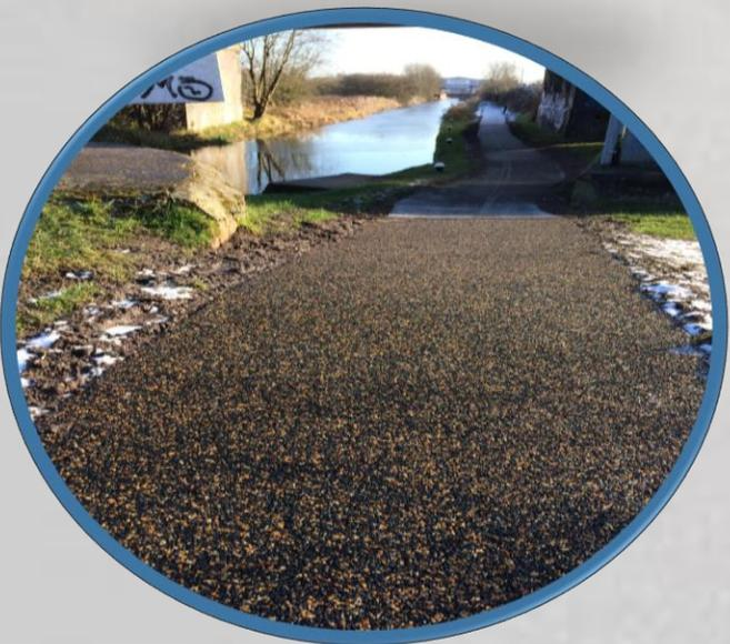
Above: The KBI Flexipave was installed on top of a simple sub-base. With a completely porous top-surface, the new path will be free from standing water and ice, creating a far more user-friendly public resource.
